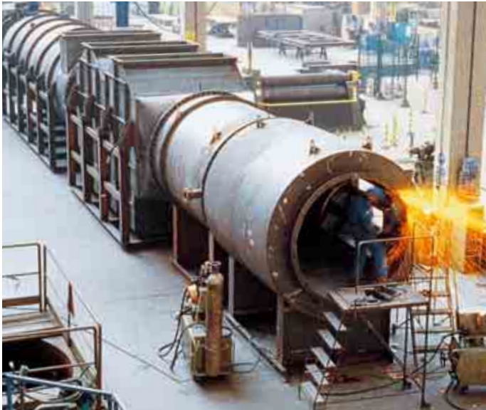
Babcock Wanson factory - Italy Recuperative oxidiser of 45,000 Nm 3 /h under construction.
