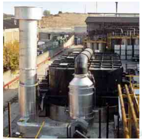
Fabric coating • 50,000 Nm 3 /h Thermal fluid heat recovery
