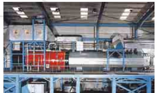
Rendering industry • Heat recovery oxidiser for steam production
